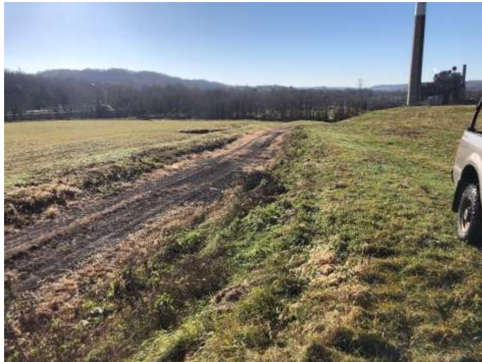
Photograph 18: Access road is well maintained.
