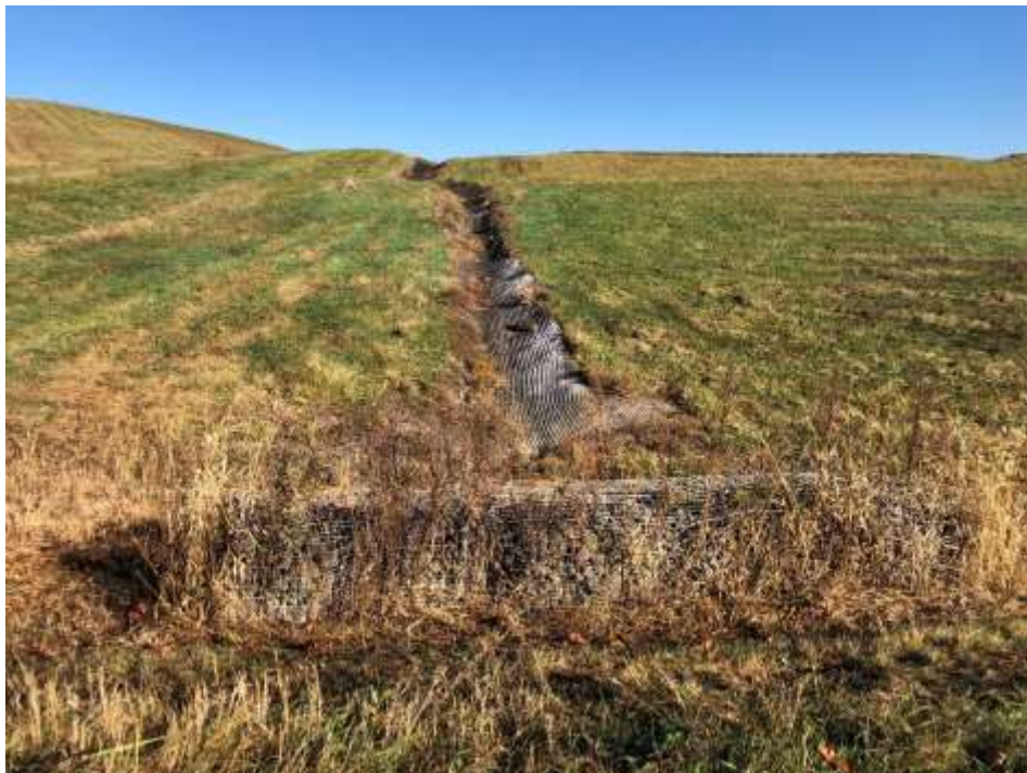
Photograph 22: Non-contact stormwater downchute is clear of obstructions. Gabion energy dissipator is installed at the junction with the stormwater (non-contact water) perimeter ditch.
