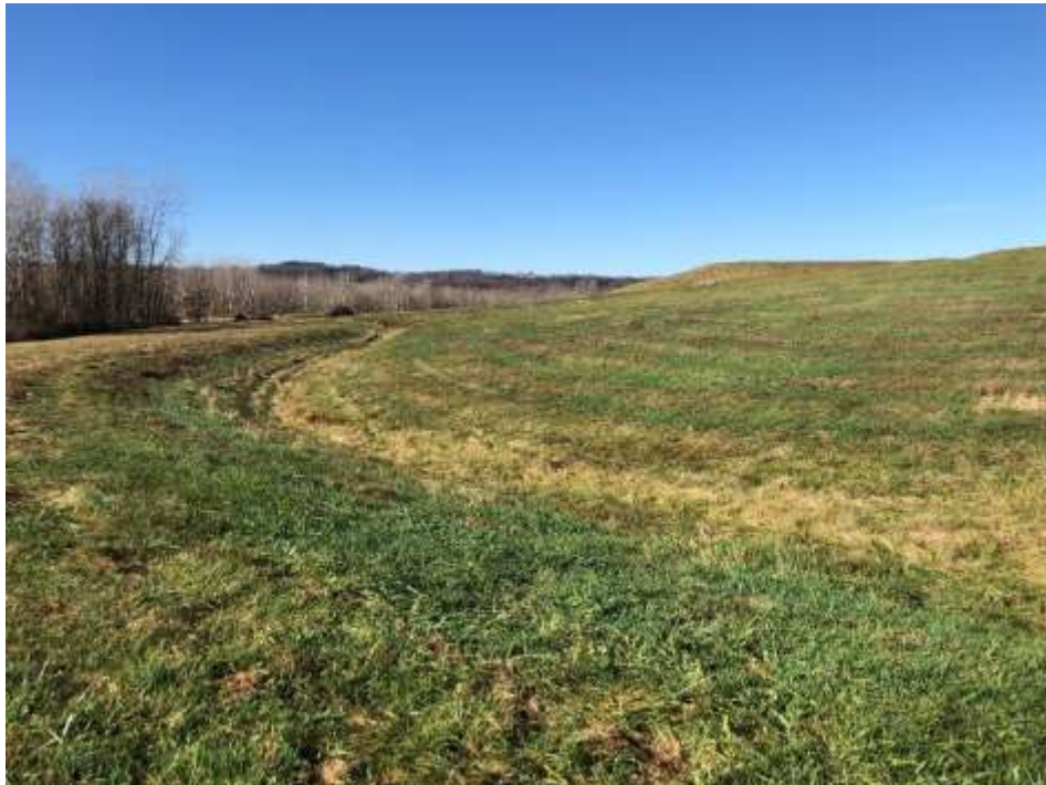
Photograph 44: South non-contact stormwater channel is clear of obstructions. South final cover lower slope is well vegetated and mowed annually. No evidence of animal burrows, erosion, or stability issues.
