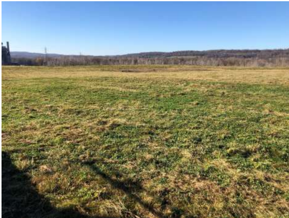
Photograph 16: Intermediate cover in active area is well vegetated and mowed annually.
