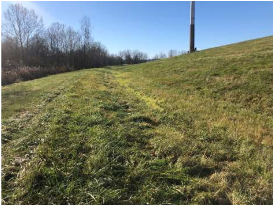
Photograph 42: East non-contact stormwater channel is clear of obstructions. East final cover lower slope is well vegetated and mowed annually. No evidence of animal burrows, erosion, or stability issues.
