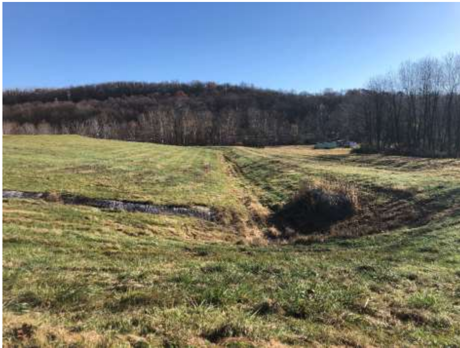
Photograph 21: South non-contact stormwater channel is clear of obstructions. South final cover lower slope is well vegetated and mowed annually. No evidence of animal burrows, erosion, or stability issues.
