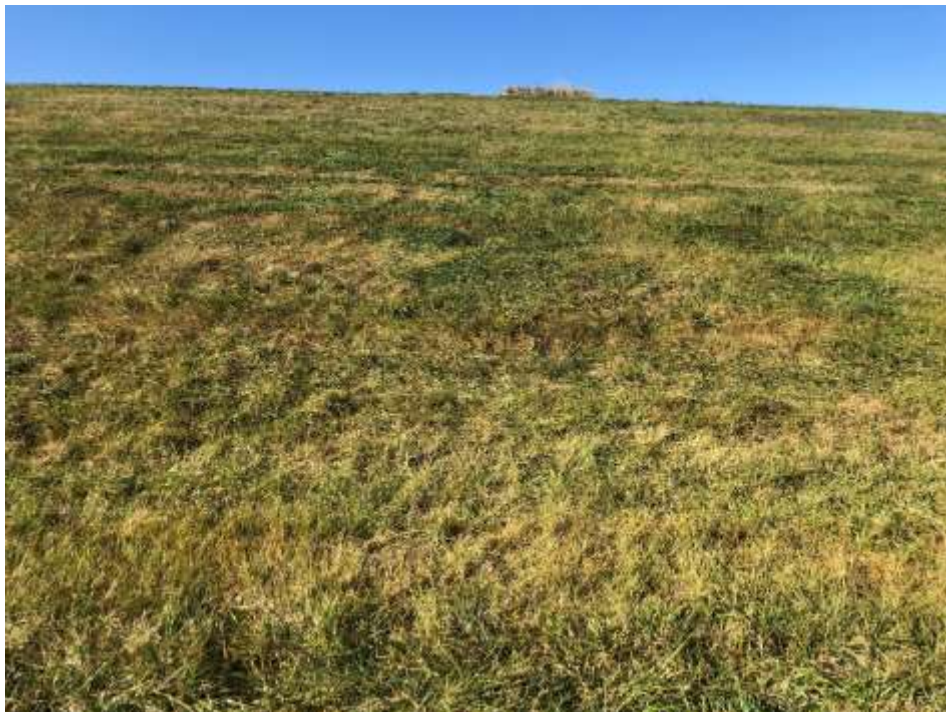
Photograph 40: East final cover lower slope is well vegetated and mowed annually. No evidence of animal burrows, erosion, or stability issues.
