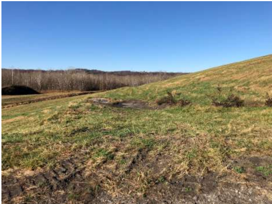
Photograph 20: South non-contact stormwater bench is clear of obstructions. South final cover upper slope is well vegetated and mowed annually. No evidence of animal burrows, erosion, or stability issues.
