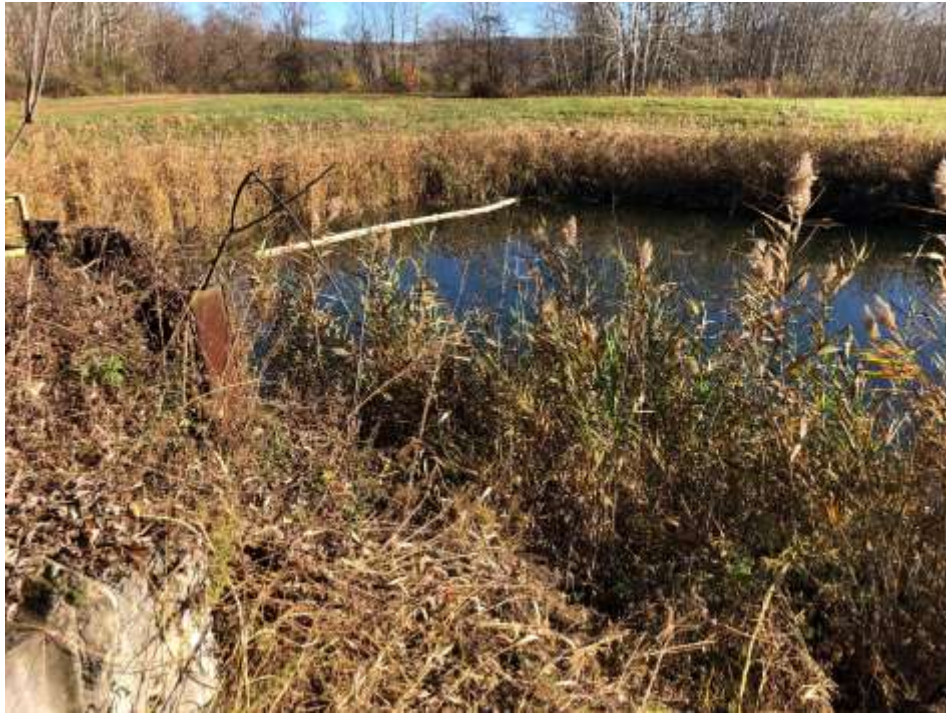
Photograph 35: Non-contact stormwater Sedimentation Pond.
