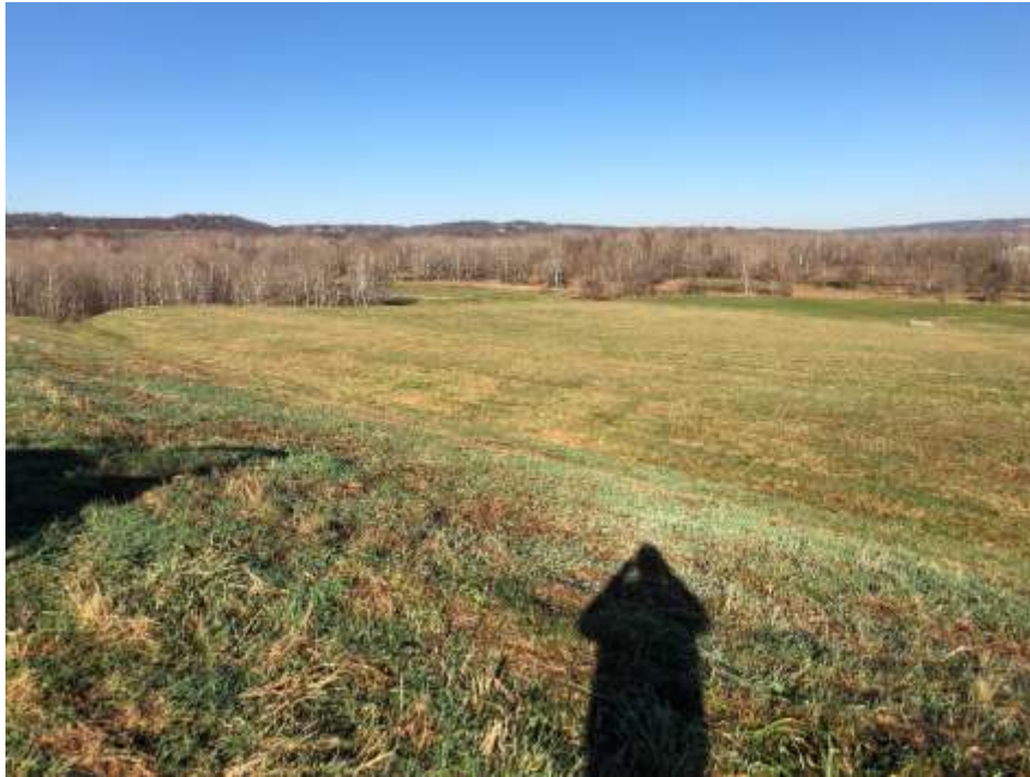
Photograph 1: Stage 5 final cover is well vegetated and mowed annually. No evidence of animal burrows, erosion, or stability issues.
