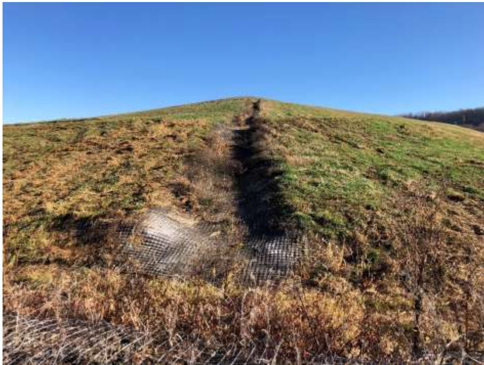
Photograph 27: Non-contact stormwater downchute is clear of obstructions. Gabion energy dissipator is installed at the junction with the stormwater perimeter ditch.
