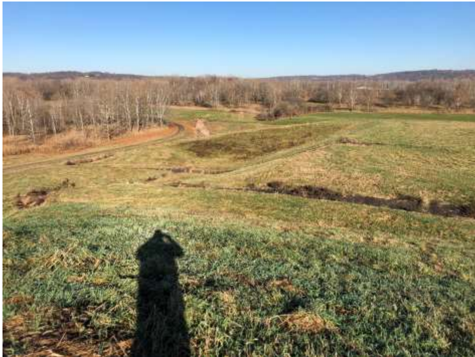
Photograph 6: Downchutes from west side of Stage 4 and Stage 5. No evidence of animal burrows, erosion, or stability issues on the vegetated slopes.
