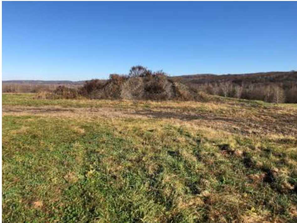
Photograph 17: Intermediate cover in active area is well vegetated and mowed annually. Bottom ash storage pile.
