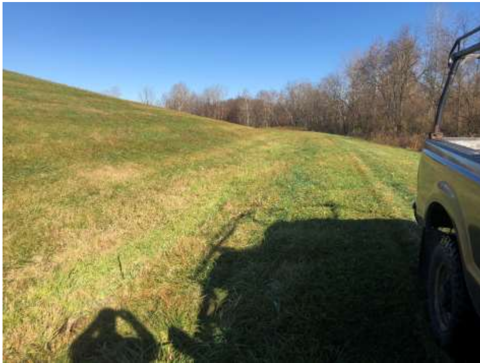
Photograph 41: East non-contact stormwater channel is clear of obstructions. East final cover lower slope is well vegetated and mowed annually. No evidence of animal burrows, erosion, or stability issues.
