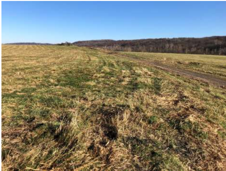
Photograph 13: Intermediate cover in active area is well vegetated and mowed annually.
