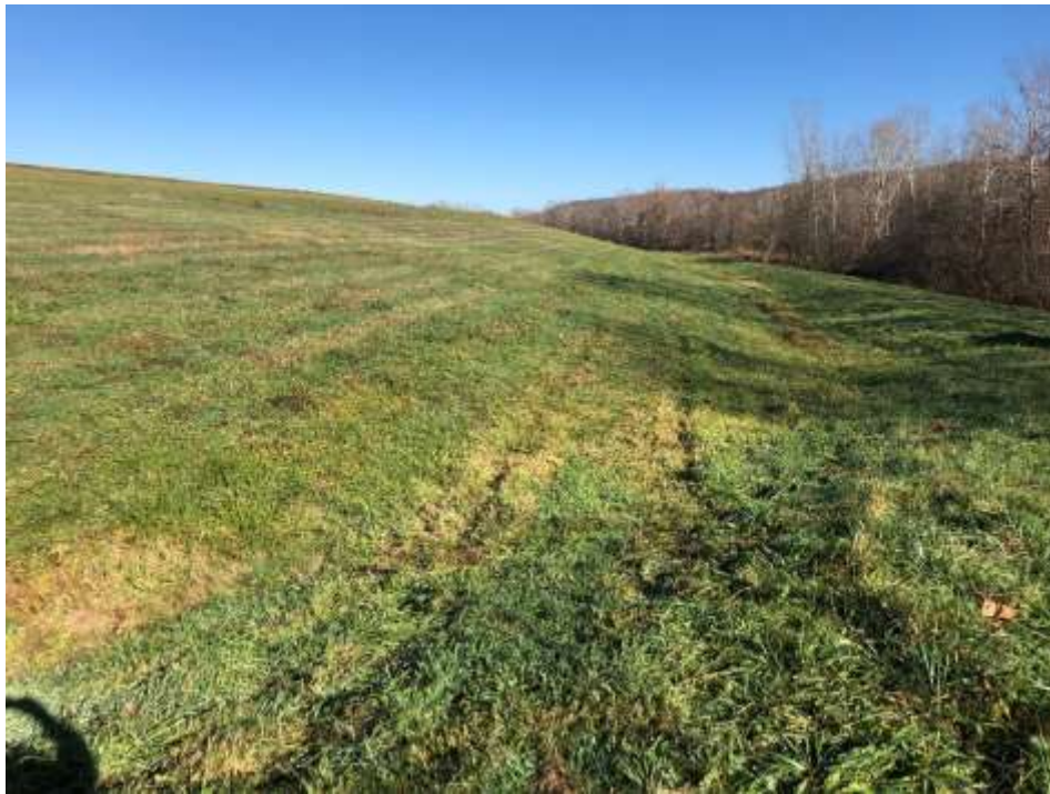
Photograph 43: East non-contact stormwater channel is clear of obstructions. East final cover lower slope is well vegetated and mowed annually. No evidence of animal burrows, erosion, or stability issues.
