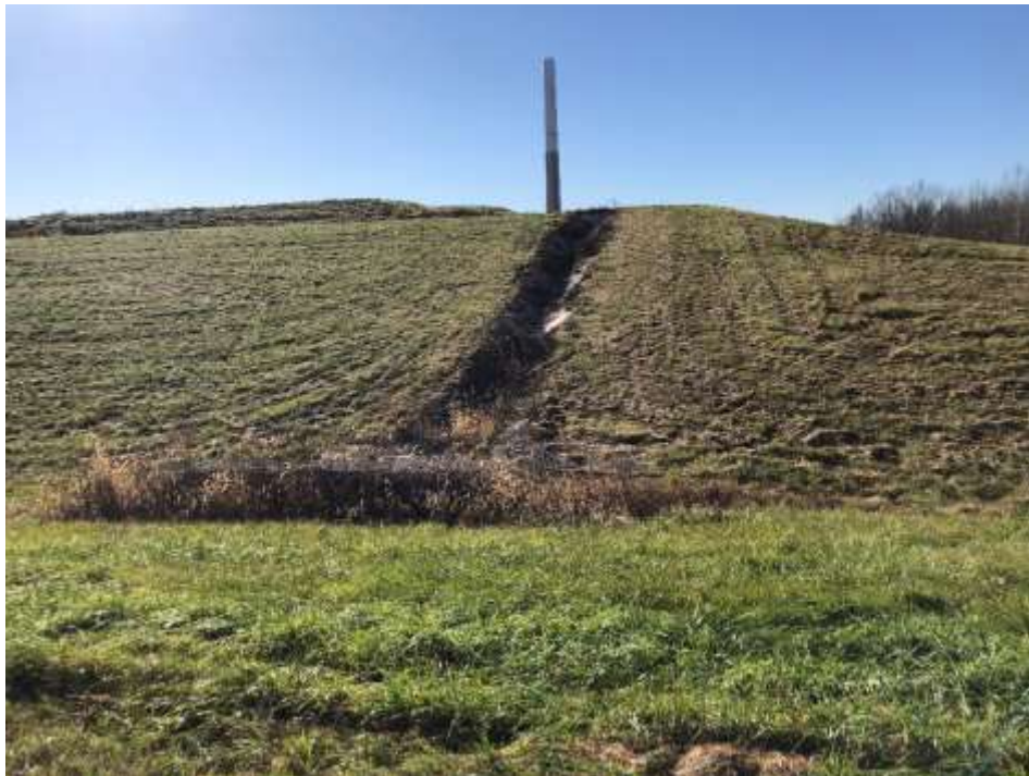
Photograph 36: Non-contact stormwater downchute is clear of obstructions. Gabion energy dissipator is installed at the junction with the stormwater (non-contact water) perimeter ditch.
