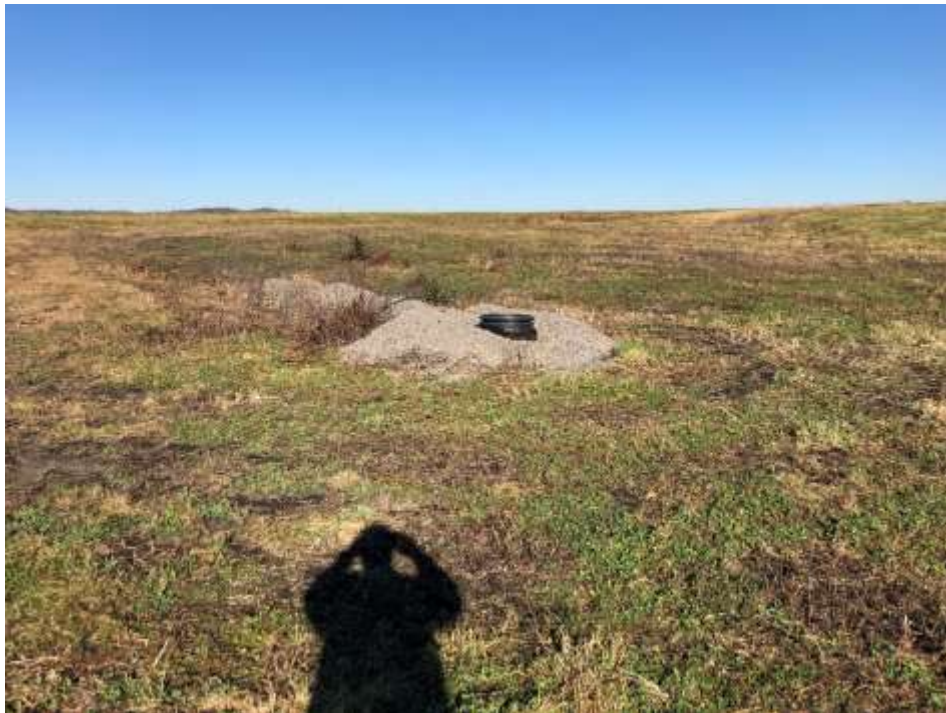
Photograph 15: Contact water collection riser in active area.
