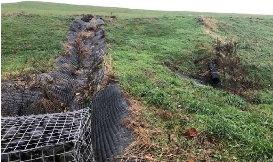
Photograph 6: Non-contact stormwater downchute is clear of obstructions. Gabion energy dissipator is installed at the junction with the stormwater (non-contact water) perimeter ditch.
