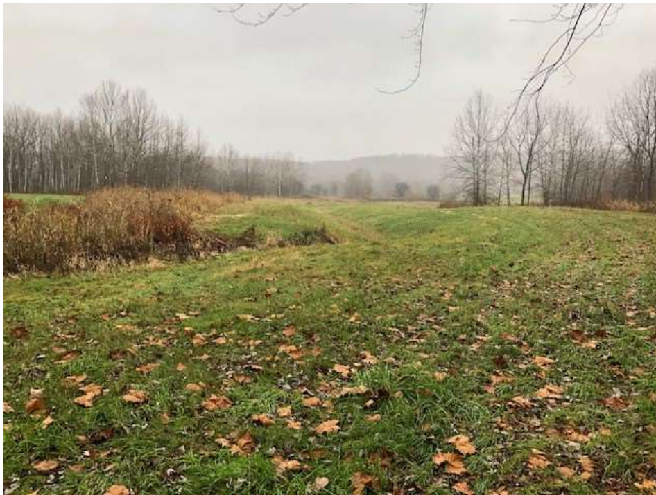
Photograph 11: North non-contact stormwater channel is clear of obstructions.
