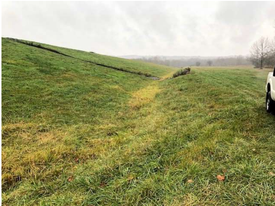
Photograph 16: North non-contact stormwater channel is clear of obstructions. North final cover lower slope is well vegetated and mowed annually. No evidence of animal burrows, erosion, or stability issues.
