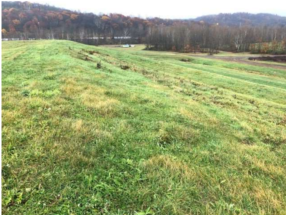
Photograph 34: Stage 4 south slope is well vegetated and mowed annually. No evidence of animal burrows, erosion, or stability issues.
