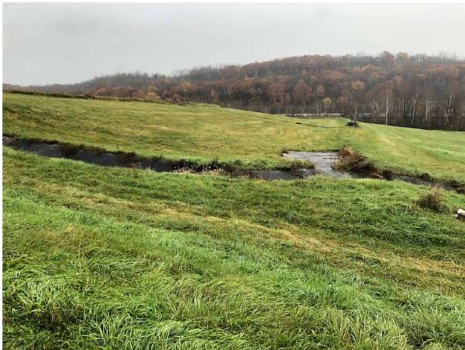
Photograph 26: South final cover upper slope is well vegetated and mowed annually. No evidence of animal burrows, erosion, or stability issues.
