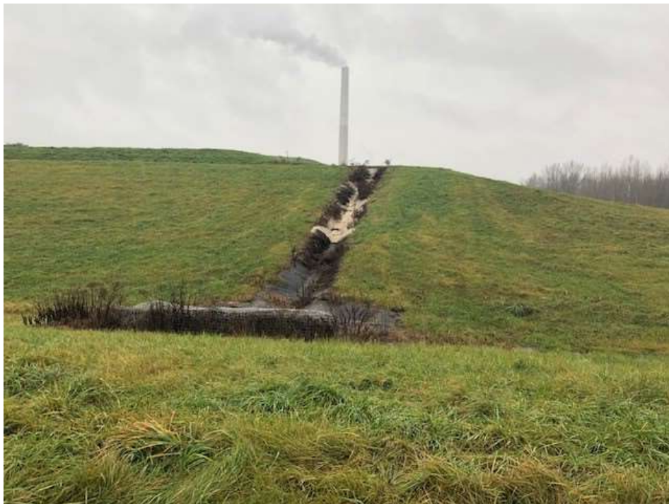
Photograph 14: Non-contact stormwater downchute is clear of obstructions. Gabion energy dissipator is installed at the junction with the stormwater (non-contact water) perimeter ditch.
