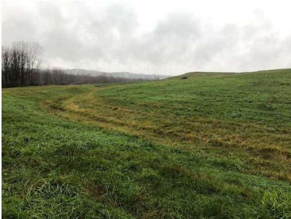
Photograph 22: South non-contact stormwater channel is clear of obstructions. South final cover lower slope is well vegetated and mowed annually. No evidence of animal burrows, erosion, or stability issues.
