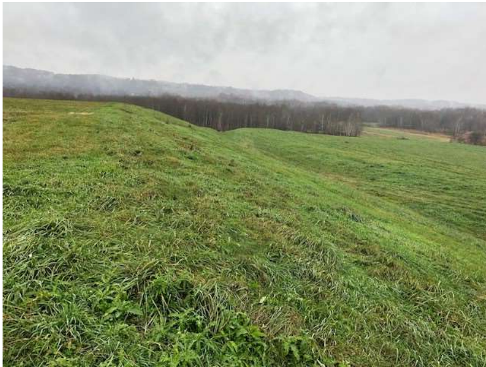
Photograph 31: Stage 4 north slope is well vegetated and mowed annually. No evidence of animal burrows, erosion, or stability issues.
