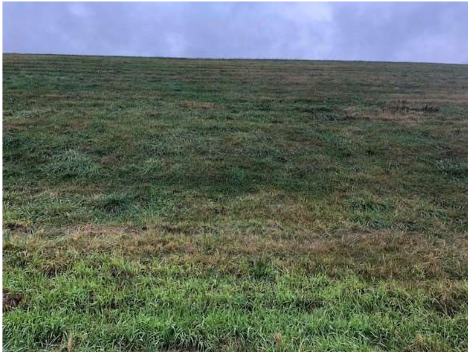
Photograph 20: East final cover lower slope is well vegetated and mowed annually. No evidence of animal burrows, erosion, or stability issues.
