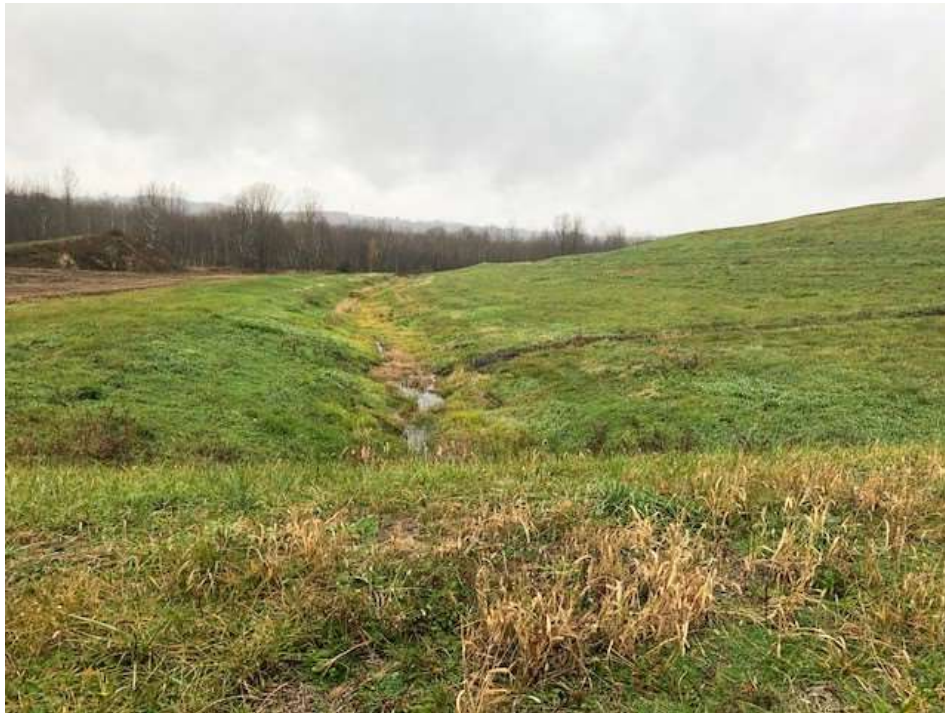
Photograph 2: South non-contact stormwater channel is clear of obstructions. South final cover lower slope is well vegetated and mowed annually. No evidence of animal burrows, erosion, or stability issues.
