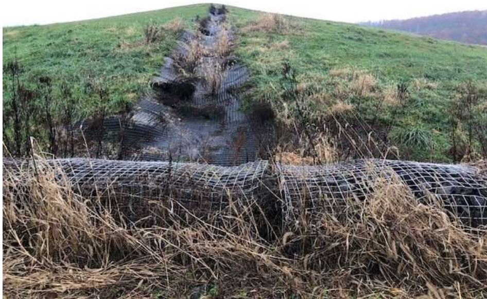
Photograph 4: Non-contact stormwater downchute is clear of obstructions. Gabion energy dissipator is installed at the junction with the stormwater (non-contact water) perimeter ditch.
