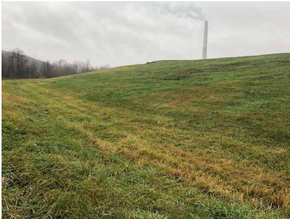
Photograph 17: East non-contact stormwater channel is clear of obstructions. East final cover lower slope is well vegetated and mowed annually. No evidence of animal burrows, erosion, or stability issues.
