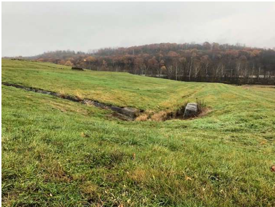
Photograph 24: South non-contact stormwater channel is clear of obstructions. South final cover lower slope is well vegetated and mowed annually. No evidence of animal burrows, erosion, or stability issues.
