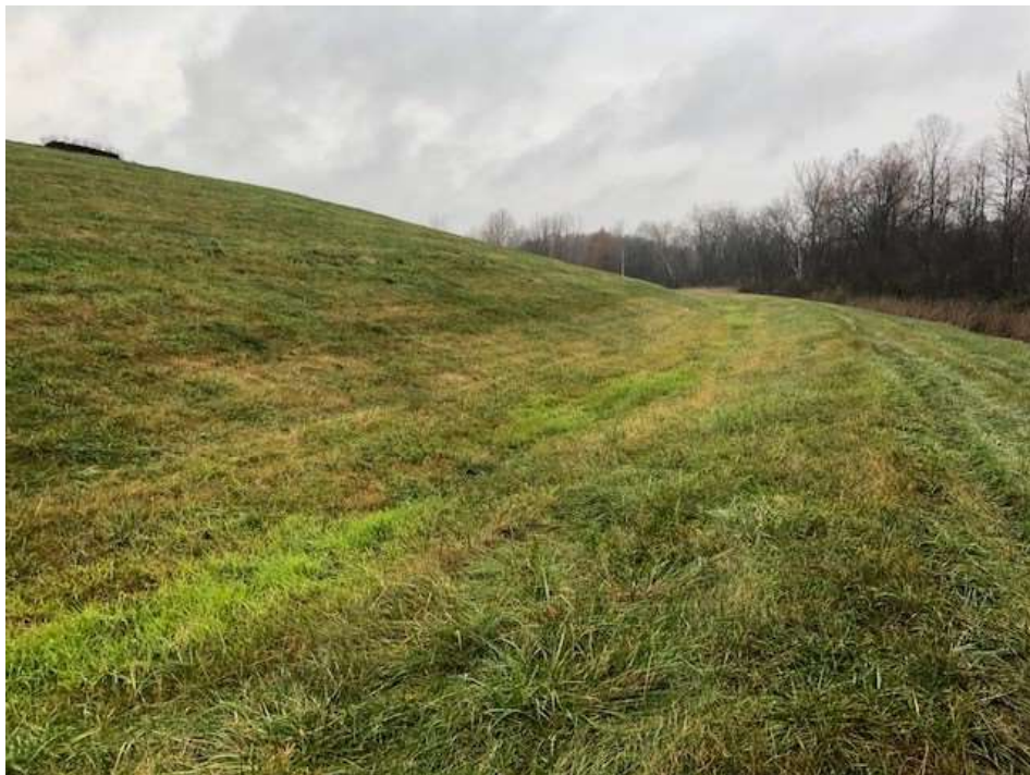
Photograph 18: East non-contact stormwater channel is clear of obstructions. East final cover lower slope is well vegetated and mowed annually. No evidence of animal burrows, erosion, or stability issues.
