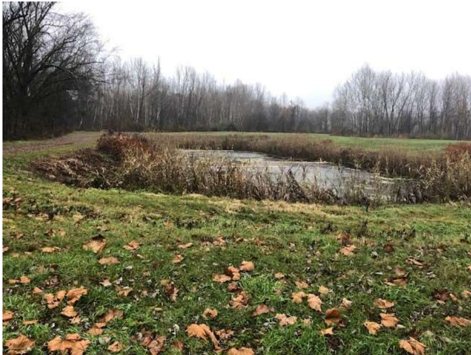
Photograph 12: Non-contact stormwater Sedimentation Pond. No evidence of animal burrows.
