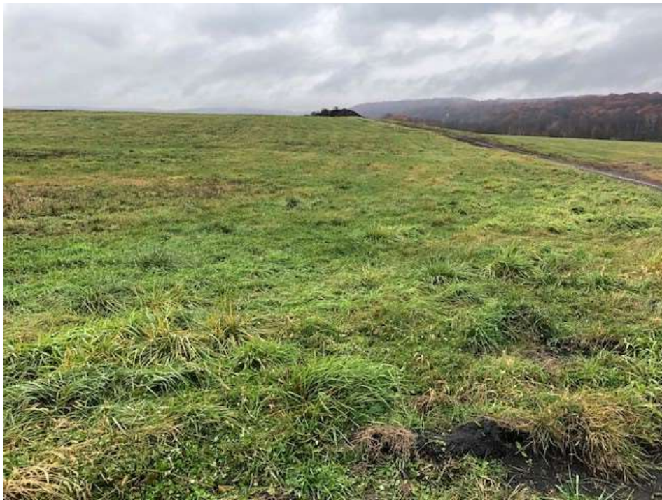
Photograph 35: Intermediate cover in active area is well vegetated and mowed annually.
