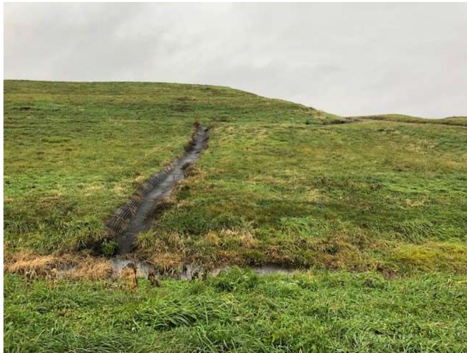
Photograph 1: Non-contact stormwater downchute is clear of obstructions.
