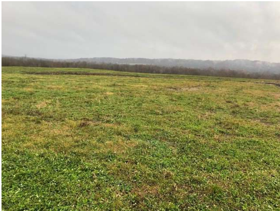
Photograph 30: Intermediate cover in active area is well vegetated and mowed annually.
