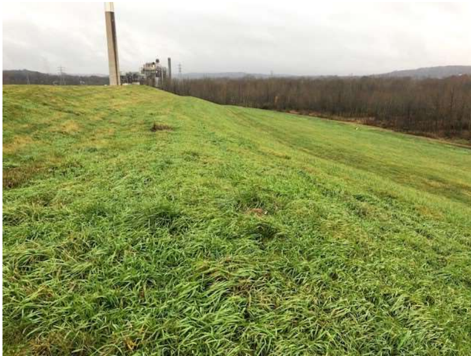
Photograph 33: Stage 4 west slope is well vegetated and mowed annually. No evidence of animal burrows, erosion, or stability issues.
