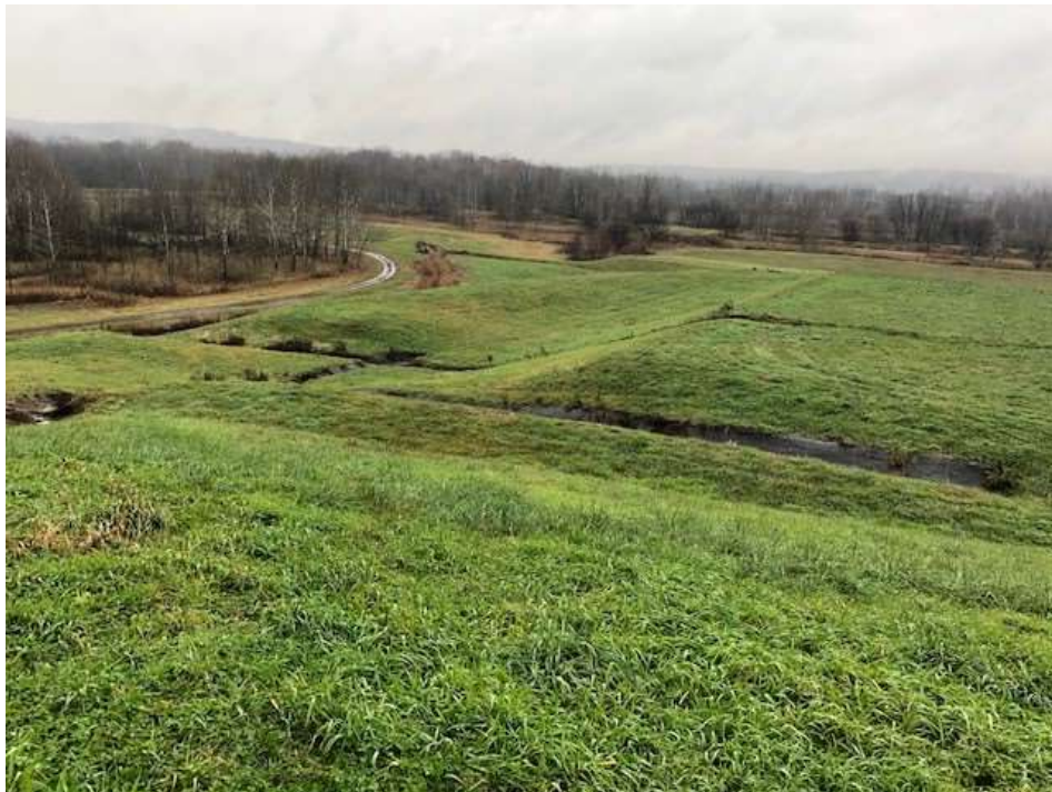
Photograph 32: Downchutes from west side of Stage 4 and Stage 5. No evidence of animal burrows, erosion, or stability issues on the vegetated slopes.
